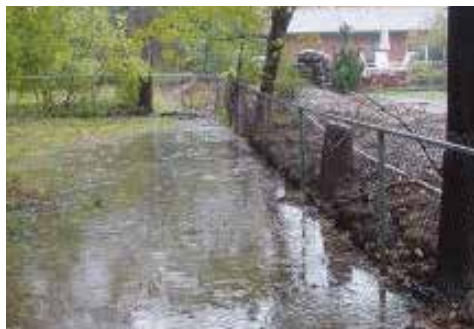
Example of Blocked Drainage Swale
